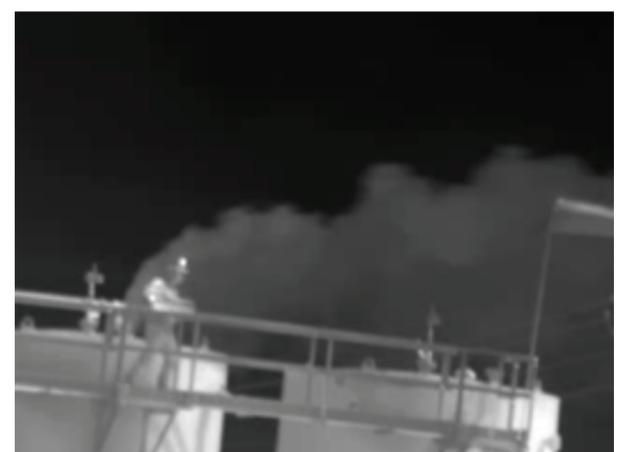
*Example: Oil and gas industry worker on tank catwalk and inside gas leak from open thief hatch.*
