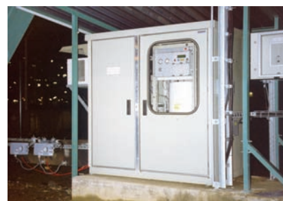
RHADOX™-system for the determination of calorific values in the flare gases of a chemical plant
