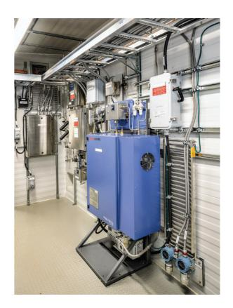
This is why a mass spectrometer was chosen for this application. A mass spectrometer uses an ionizer to convert the sample into ions, the detector then calculates the mass of each ion and langes to the system.
