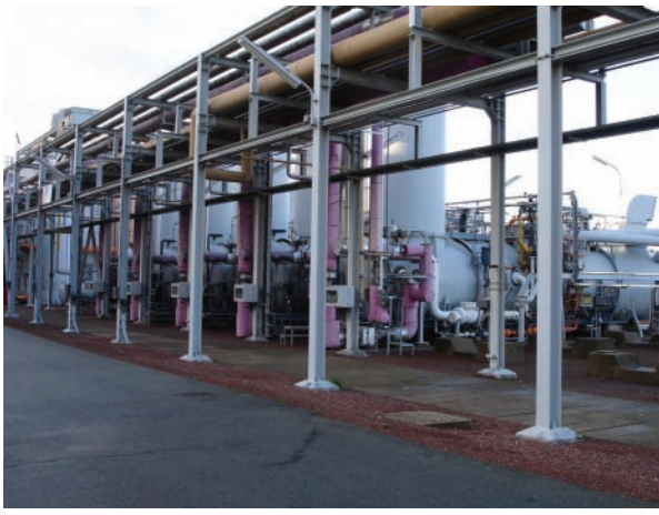
Picture 5: The instruments are installed in a hazardous environment zone 2. Therefore they are equipped with an EExd housing.
