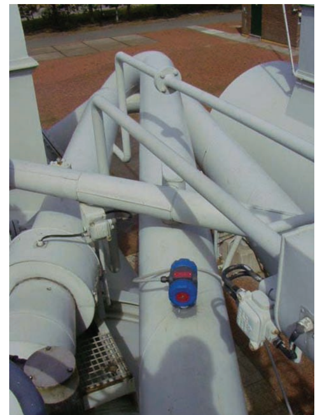
Picture 4: The Thermatel TA2 is based upon thermal mass flow measurement
