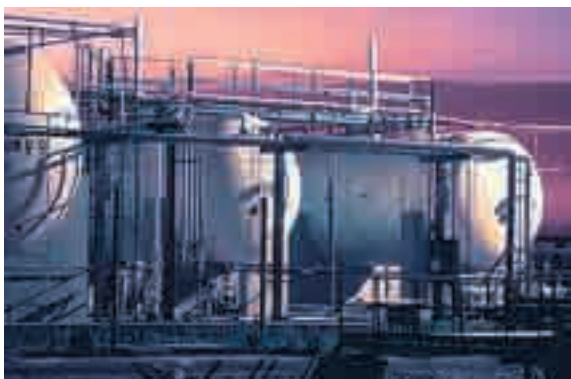
Figure 1. Typical Oil Refinery Operation
