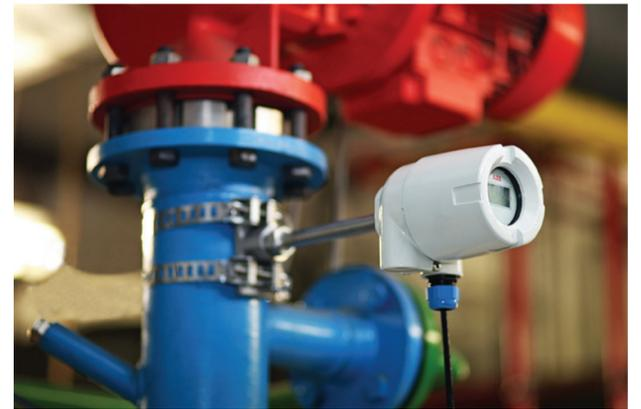
be the first step towards eliminating the need for a thermowell in future plants. However, as with any new approach, its performance will need to be carefully validated by operators and engineers the world over. At present, there are over 80 global players in the chemical, oil and gas, pulp and paper, power, food and beverage and wastewater industries that are validating the performance of our technology against existing thermowells.
