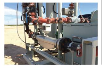
Commercially introduced in the 1980s, Coriolis mass flowmeters have become one of the most versatile and reliable means of measuring the flow of liquids or gases. Their main strength is in their ability to measure multiple attributes over sustained periods with high repeatability and very little maintenance.
